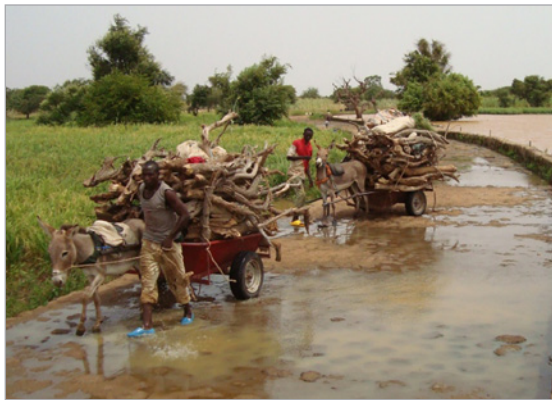
Figure 3: A water-spreading weir designed as a ford for crossing the valley. Source: Bender (2011), S. 16
