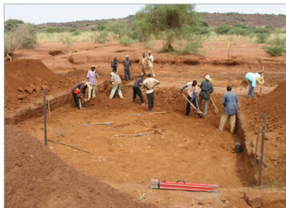
Figure 7: Training site for local craftsmen. Source: Lütjen
