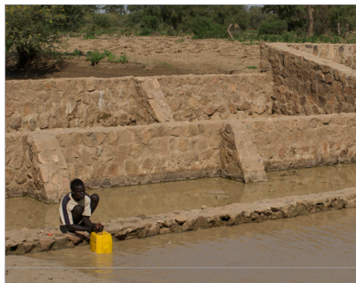
Stagnant water in water-spreading weir
