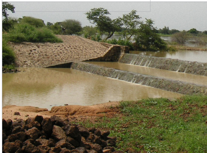
Water-spreading weir in Kalfou (Tahoua region, Niger)
